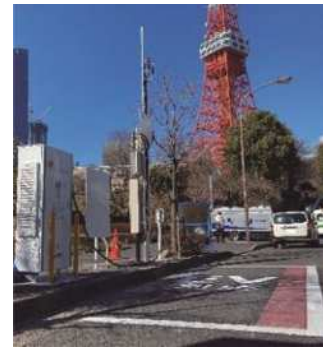
A charger installed along a public road in an area with parking meters
