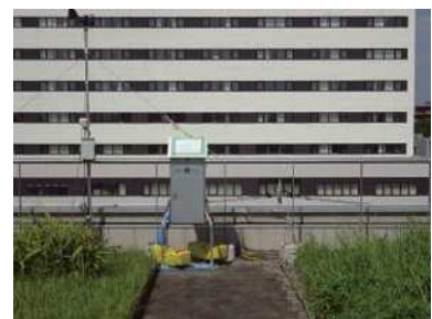
View of monitoring equipment
