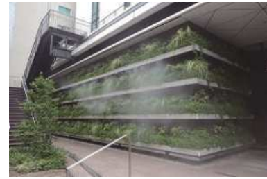
Example of installation of fine misting devices (OASE Shibaura, Minato-ku)
