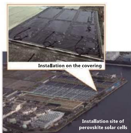
Morigasaki Water Reclamation Center
