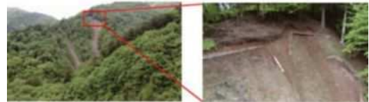
Using drones for on-site investigations
