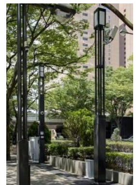
Smart pole with 5G base stations in Nishi-Shinjuku
