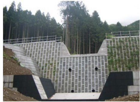
Erosion control facility
