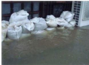
Protecting chemical substances from immersion: Installation of sandbags
