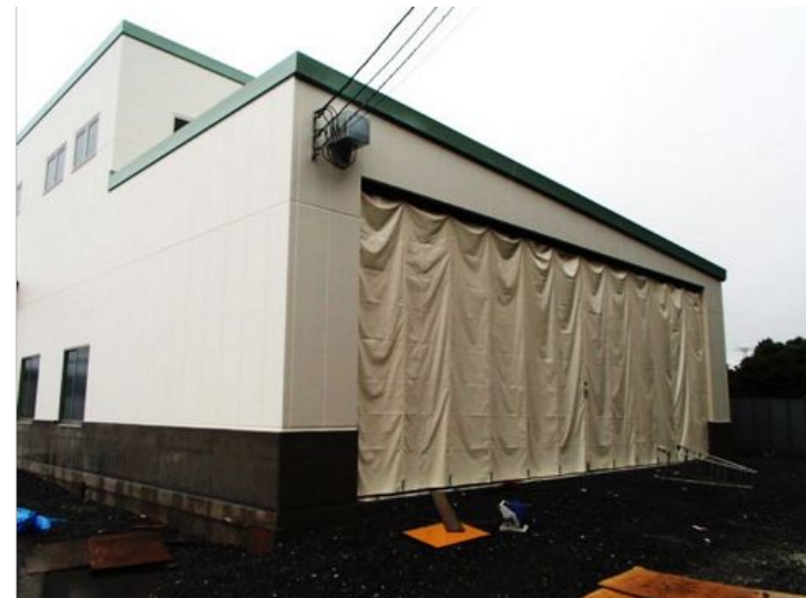
入庫パネル保管棟(右側)
