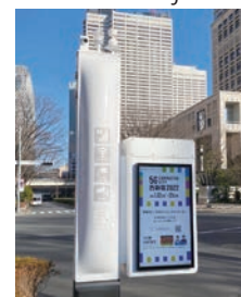
Smart pole with 5G base stations in Nishi-Shinjuku
