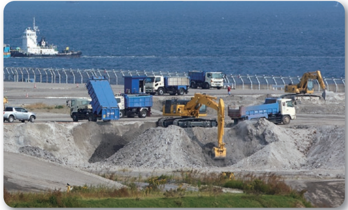
At present: Intermediate processing is carried out before landfilling—garbage is burned and incombustible waste is pulverized.
