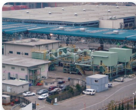
Facility for pulverizing bulky waste
