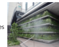
Installation of fine misting (OASE Shibaura, Minato City)
