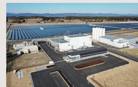
Fukushima Hydrogen Energy Research Field (New Energy and Industrial Technology Development Organization)
